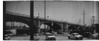
10P3 LA State Historic Park-Bridge_2nd Workshop 2011.jpg (2013.749)
